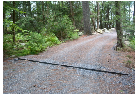
A rubber razor on a well-maintained camp road helps divert rainfall into ditches and forested areas.
