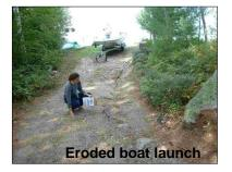
Due to the nature of their design and purpose, boat launches also tend to direct runoff into lakes. Typical problems observed on boat launches in watershed surveys include surface erosion, poor surface material and shoreline erosion. Even lakes with public boat launches commonly have several, if not dozens, of private launches.
