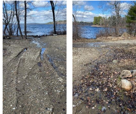
Site JS-5 (left) and site JS-6 (right) – stormwater runoff entry points.
