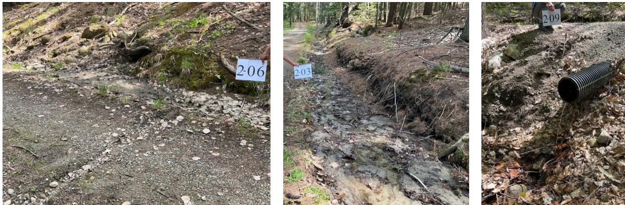
Erosion sites identified on Dole's Beach Road / The Boulevard in Sector 2. Runoff over-topping the road (Site 2-06) and eroding a channel in the road surface, and overwhelmed ditch full of sediment that drains to Androscoggin Lake (Site 2-03), and an unstable culvert outlet (Site 2-09).
