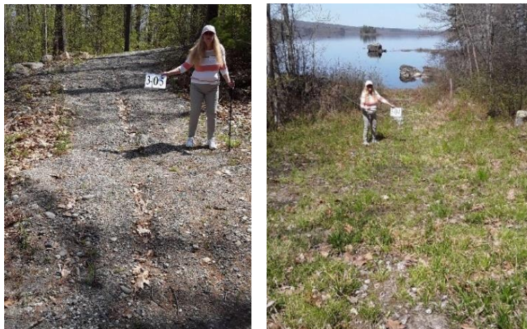
Site 3-05 (left) and site 3-04 (right) identified on Moose Run Road in Sector 3.
