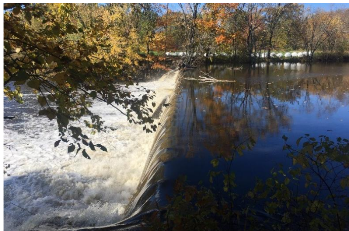
The Dead River pollution control facility in October 2021 ( top) and flow reversal in October 2022 after heavy rains caused the Androscoggin River to rise ~16 feet (bottom).
