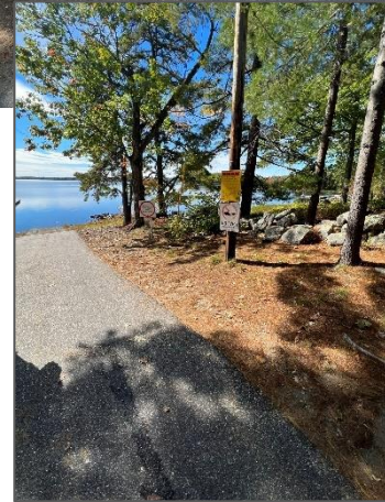
Erosion at roof driplines and adjacent common spaces (top) and boat launch (bottom) documented at site 9-14 in Wayne
