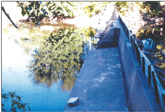
Dead River Dam with 2-foot flashboards.
